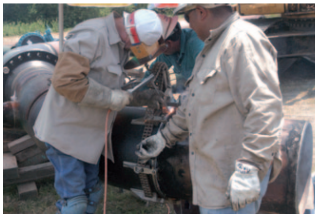
FIGURE 2-18 Welders and welding helpers must wear appropriate general work clothing.
