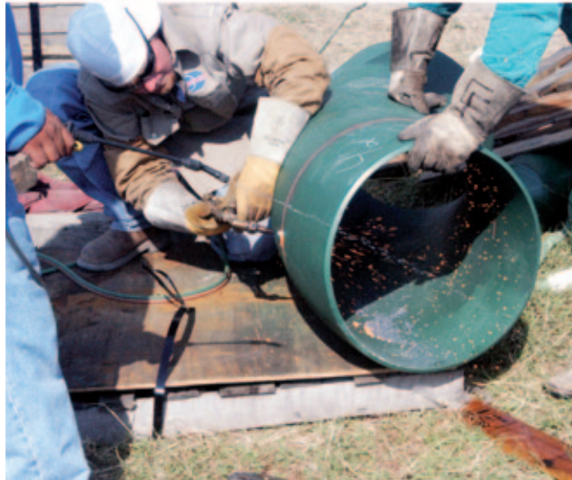
FIGURE 1-24 Plywood used to protect dry grass from the sparks given off from the cutting torch.
