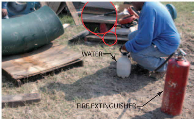
FIGURE 2-20 A fire watch has both a water sprayer and a fire extinguisher. A fire safety officer does not have to see a fire happen; the burned grass on a site may be enough to shut down welding.
