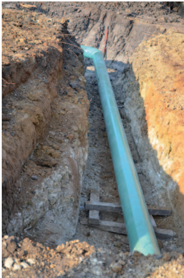
FIGURE 2-15 Example of benching (on the left wall) and sloping (on the right wall).
