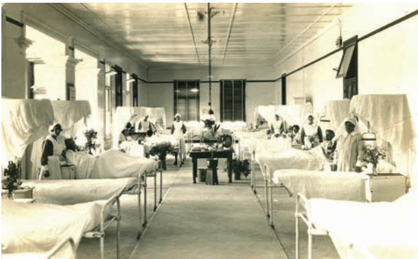
FIGURE 1-2a Male medical ward, Ipswich Central Hospital, Queensland, 1927
