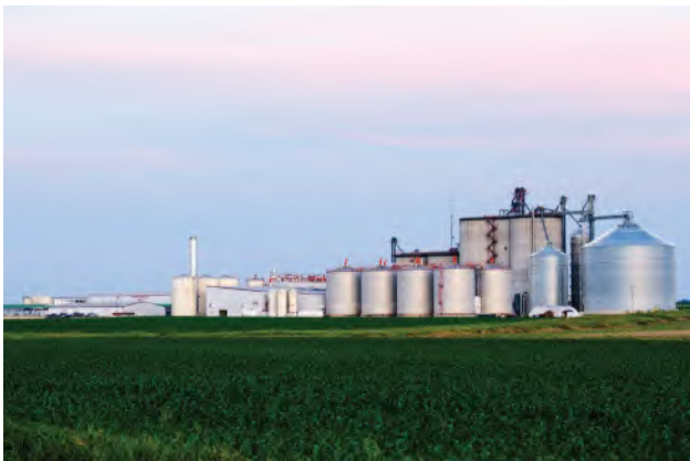
Fig. 1-1 Use of natural energy sources (green energy) such as solar, wind turbines, and bio-fuels like ethanol are getting a tremendous amount of interest in the way of research, development, and real applications. As they continue to develop, other issues will need to be dealt with, such as ROI. Welding plays a very important role in the manufacture of these green energy sources. (top) Stocktrek Images/Getty Images; (middle) Bear Dancer Studios/Mark Dierker; (bottom) Mark A. Dierker/McGraw Hill
